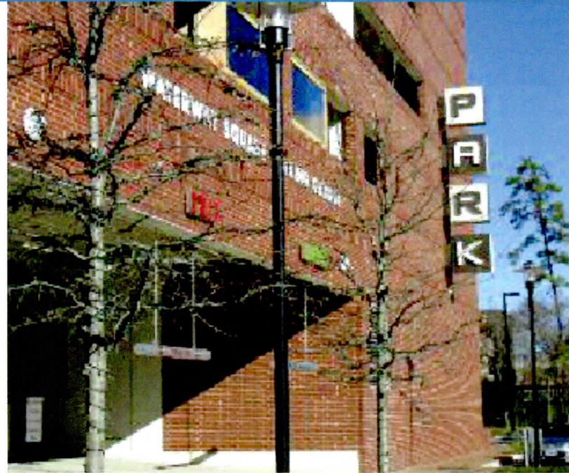
Parking entrances are off the main pedestrian area at the Woodlands.
